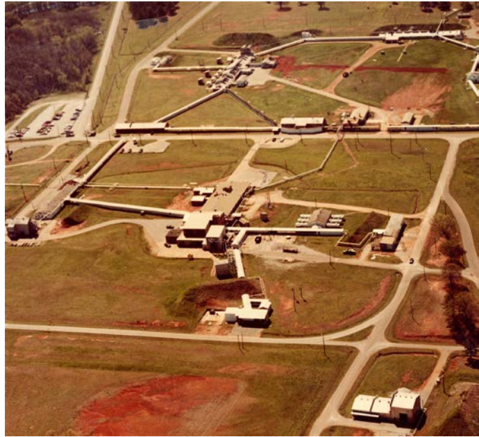
Figure 25. Sidewinder/Mk 70 facility looking south.
