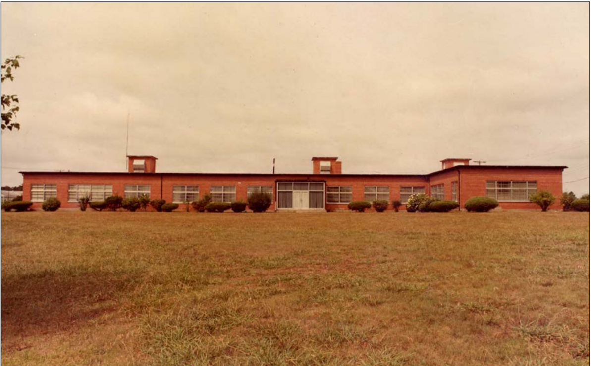
Figure 2. Administration Building (7650), looking west from Line Road.
