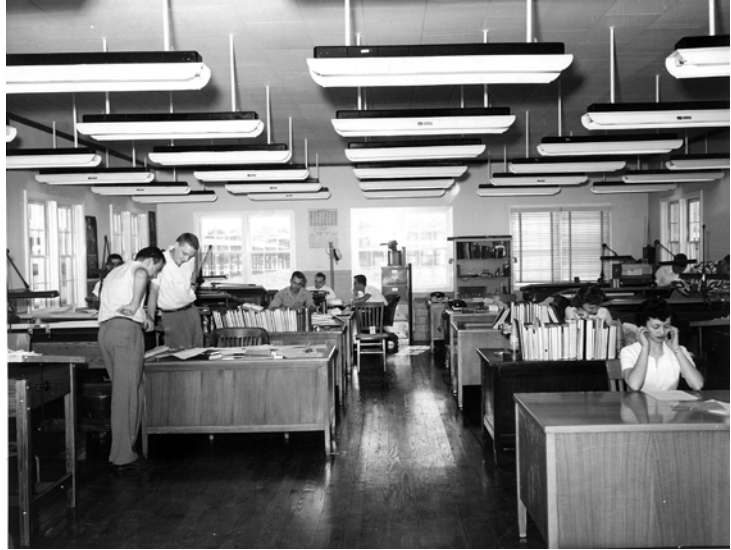
Figure 3. Inside the Engineering Building (7631) in 1951.
