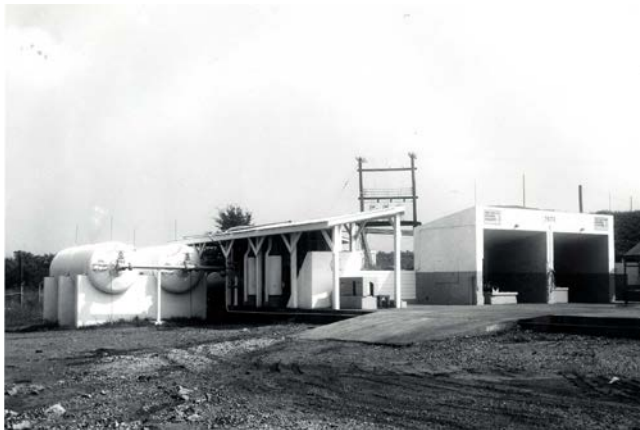
Figure 30. Original Direct Connect Facility (1966).
