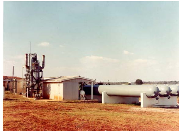
Figure 31. Direct Connect Facility Upgrade.
